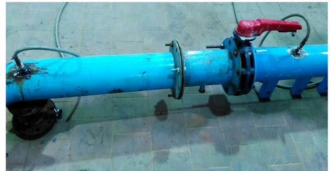
**Fig. 3** :Arrangement of taps pressure upstream and downstream the UPVC butterfly valve.
